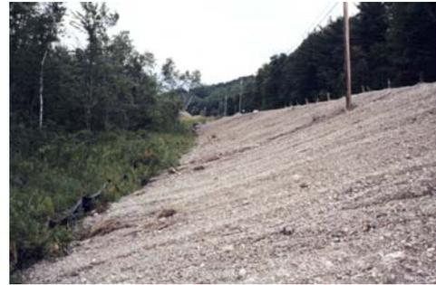
project that required building a newly constructed 1:2 slope that was adjacent to a wetland. The proximity of the site to the wetland required immediate erosion control. It was decided by the EAD and the AOT, that the site would be an excellent demonstration for compost erosion control mulch.
