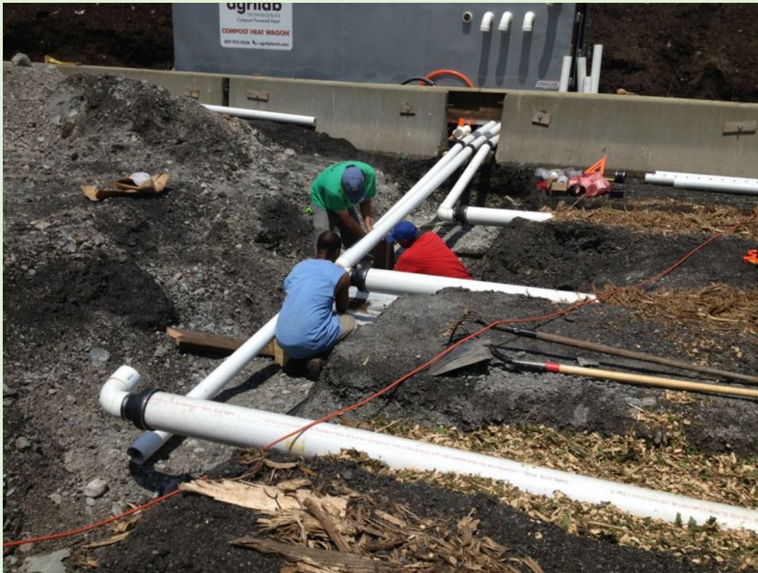
Aeration Pipe Assembly in Boston
